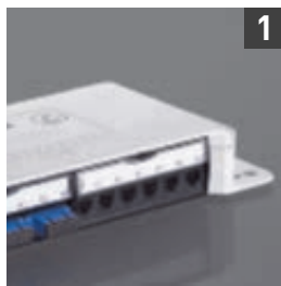
Area distribution box
