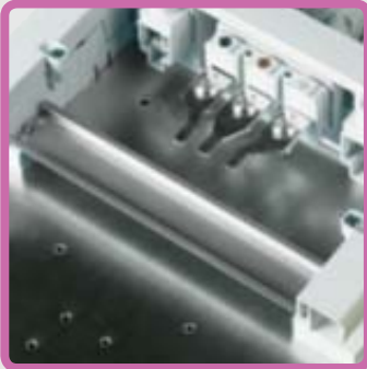
Step 2: Fitting the terminals at the end of the busbar.
