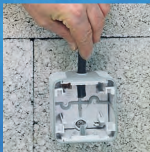
2/ Insert the cable through the end cap
