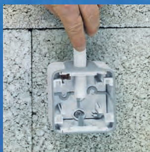
2/ Insert the tube through the end cap
