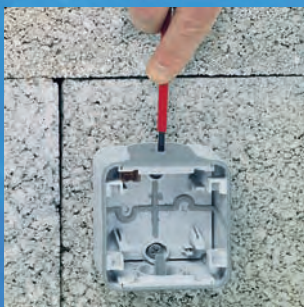
1/ Pierce the end cap using a screwdriver
